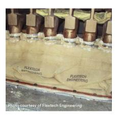
Tube seals mounted while the furnace is in the cold or contracted condition. When the furnace comes to temperature, the tubes will expand and put pressure on the seals. maintain their shape in environments like process heaters and furnace reformers while helping to prevent the formation of harmful emissions. Because they are flame resistant, they are also a safety measure against potentially damaging flames from a draft fan failure.
