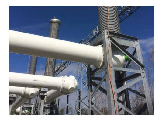
After four years' research, GE, using 3M<sup>™</sup> Novec<sup>™</sup> 4710 Dielectric Fluid has developed an SF<sub>6</sub>-free solution that is much more environmentally sustainable yet meets all the very tough specifications for HV switchgear, including high dielectric strength, good arc quenching capability, compatibility and easy handling.
